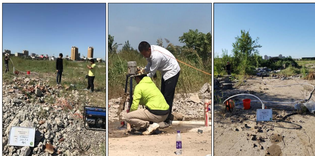
图 6-7 螺杆自吸泵洗井
